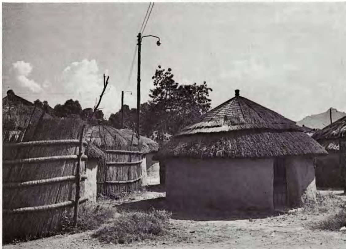
Street Lighting in Swaziland! A typical example of rural electrification at the village of Lobamba.
