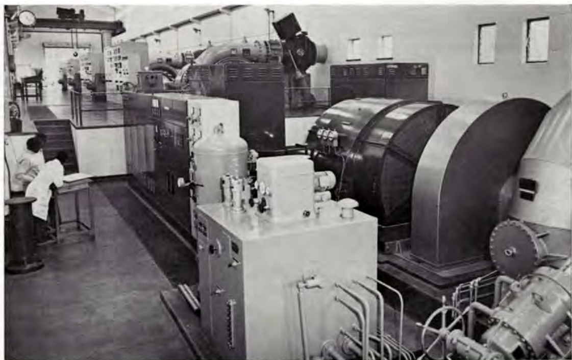
A general view inside Edwaleni hydro generating station turbine hall.
